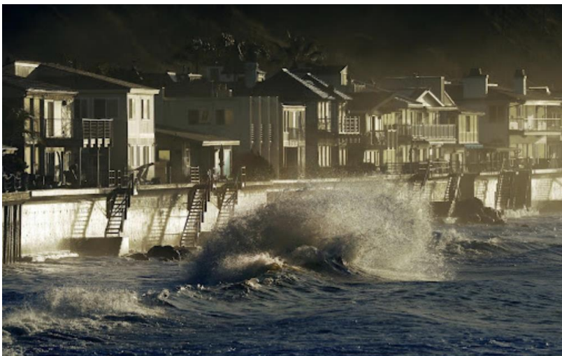
Seawall in Ventura County, California. Credit: Al Seib/Los Angeles Times
